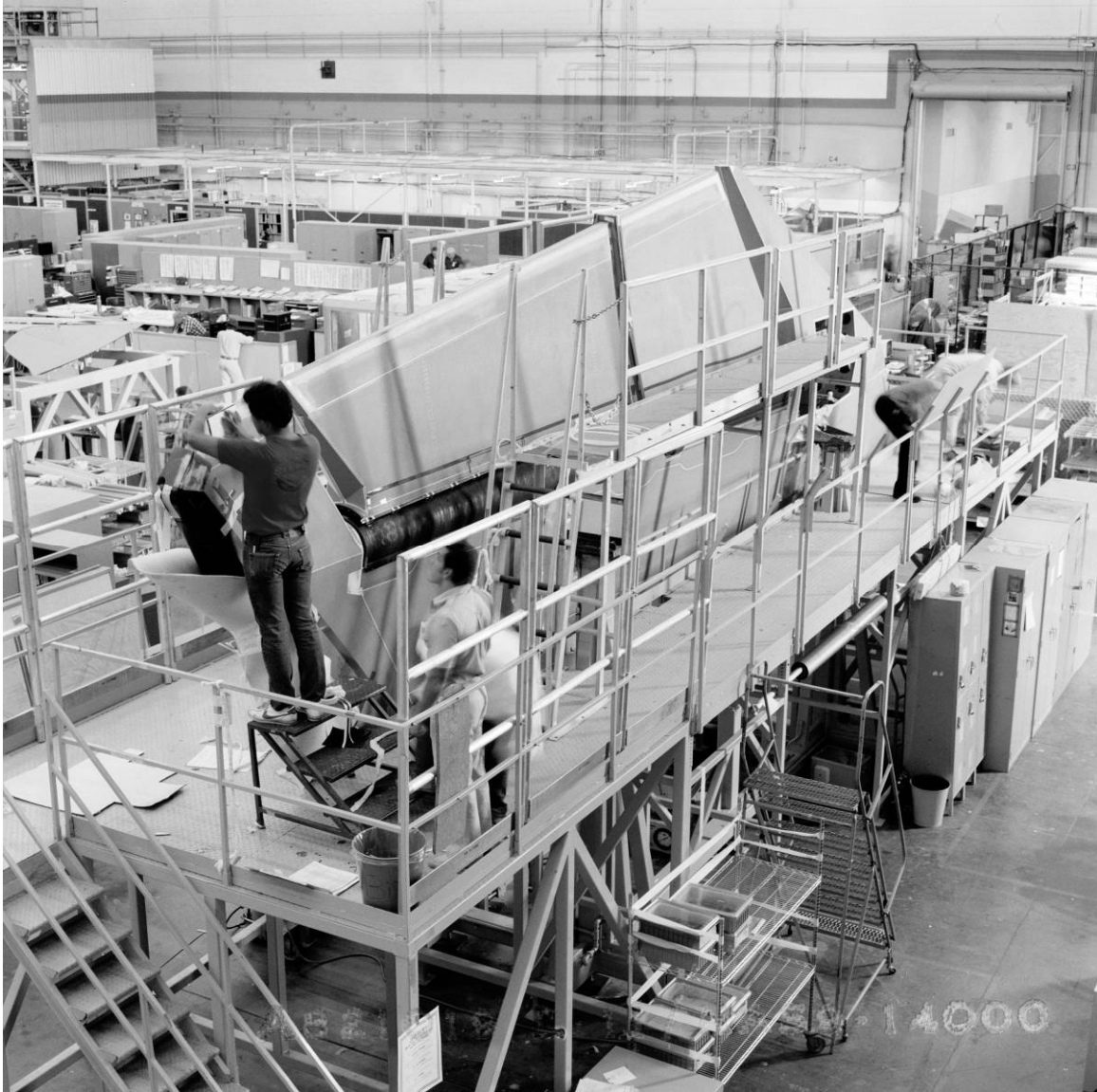
Figure B-30. Installation of TPS on Discovery's vertical stabilizer, AFP 42, October 19, 1982. Source: NASA, Johnson Space Center Image Repository, JSC2010-03353.
